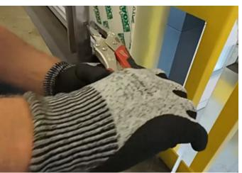
13. Once the extrusions are notched, clamp the extrusion onto the end of the rails and fasten using a self-drilling fastener into the deep return of the extrusion. This process will be similar with both a corner extrusion and termination extrusion.
