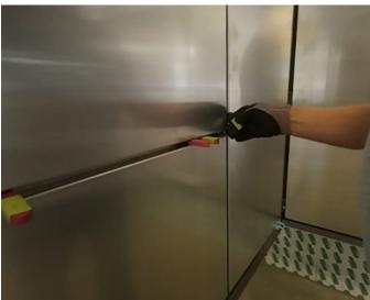
8. Use shims to achieve the appropriate panel spacing along both the horizontal and vertical joints. When shimming the horizontal joint, it is necessary to ensure there is a 5 mm gap between bottom of the hook and the rail to allow for thermal movement.
