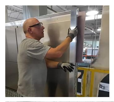
16. Finally, snap on the appropriate extrusion caps at the termination and outside corner locations, using a rubber mallet as needed.
