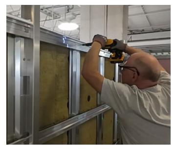
6. Fasten the rails into the subgirts through the predrilled holes. When the first set of rails are fastened, remove the jigs and set them up further up the wall. This can be used as a guide to set up the next few rows of rails. Repeat this process until all the rails are set up.
