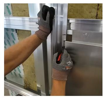
11. When you get to an outside corner or end detail, you must prepare the female extrusions by creating a 3" notch on the receiver legs wherever there is a horizontal joint in the panel to allow the female extrusion to continuously run through the wall.
