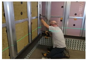
3. Once the jigs are aligned and level, temporarily fasten the jigs to the subgirt.
