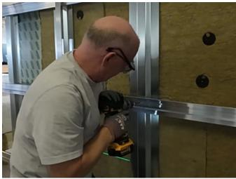
5. When rails are in place predrill holes into the rails at required project spacing.
