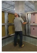
7. If there is an inside corner always start the installation from the inside outwards. Otherwise, it is recommended to install from left to right. Hook the panels onto the rail to align the top of panel with the bottom lip of the rail that the panel is attached to.
