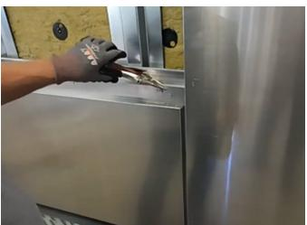
10. Repeat the process along the wall, ensuring that all panels are appropriately shimmed and fastened correctly to the rail. During the installation of the panels, it is necessary to install a cover plate at any intersecting panel joints throughout the elevation. These plates are simply fastened with a self-drilling fastener.
