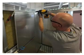
When aligned, clamp the panel in place and fasten the panel to the rail using the pre punched holes along the top flange as a guide.
