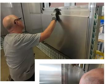
15. Hook the cut panels onto the rail and clamp the cut side of the panel onto the extrusion. Ensure the panel is shimmed correctly along the horizontal and vertical joints. Once the panel is in place fasten the cut end of the panel into the leg of the extrusion and fasten along the top flange of the panel in the pre punched holes.
