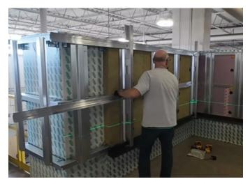
4. When the jigs are fastened, feed the rails through the jig openings at the pre-determined project spacing.
