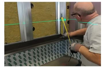
2. First, align the Jigs so the bottom the jig is lined up with the bottom of the first row of panels. Set up a laser level to a datum line that can be referenced when fastening.
