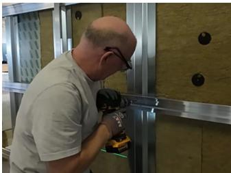
5. When rails are in place predrill holes into the subgirt at required project spacing.
